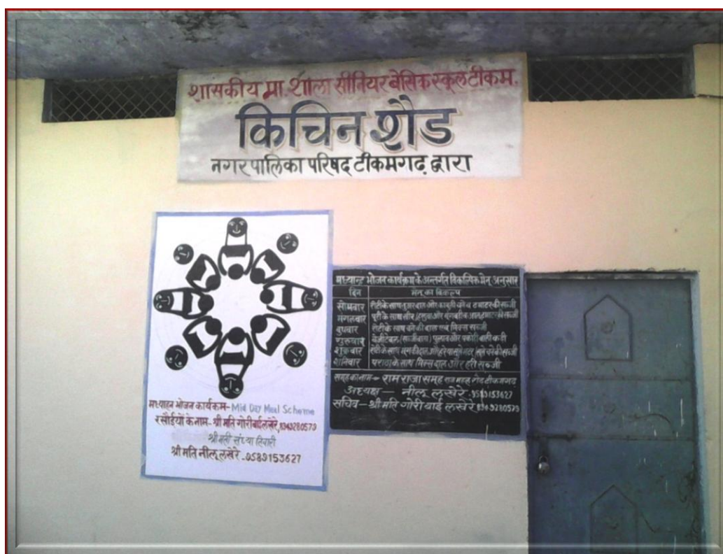
Condition of kitchen Shed
